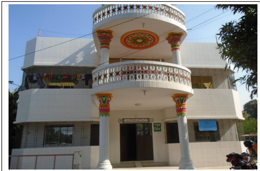
Picture-6.3: Field Office at Dohar
