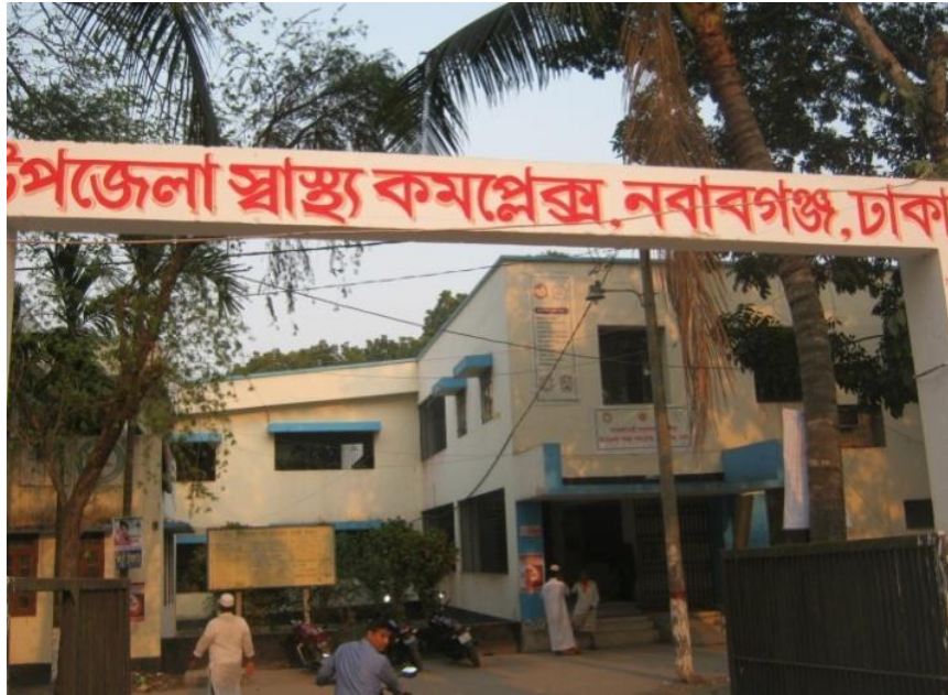
Picture 2.5: Nawabganj Upazila Health Complex
