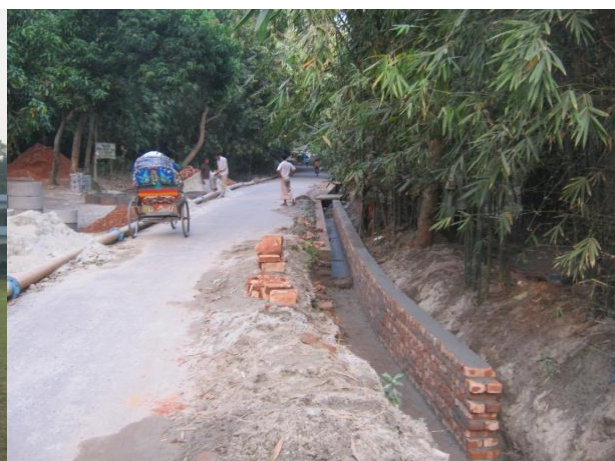
Picture 2.4: Urban Drainage Facility under Construction.
