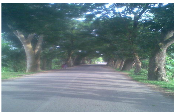
Picture 2.8: An Arterial Road in the Shibchar Upazila
