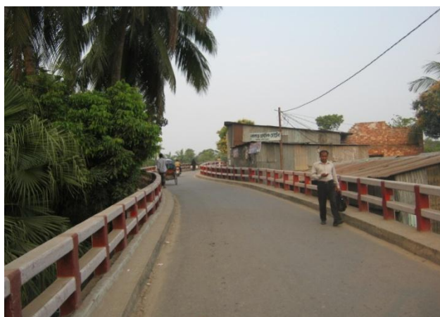
Picture 2.1: Nawabganj Ichamati Bridge
